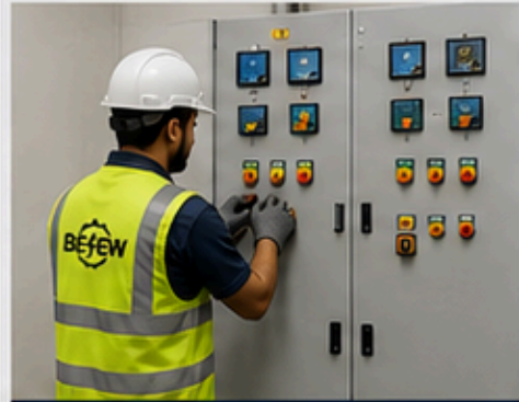
PCC PANEL INSTALLATION
