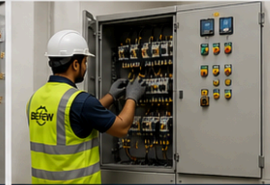
AMF PANEL INSTALLATION
