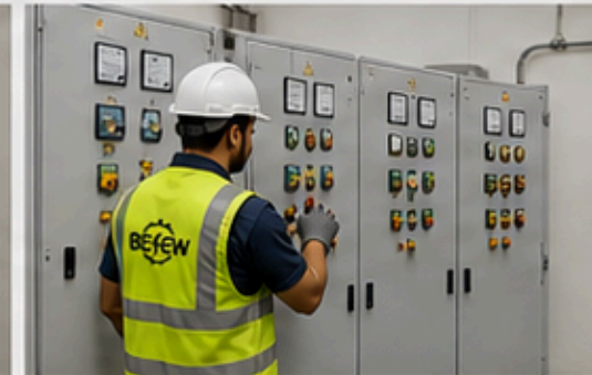
HT PANEL INSTALLATION
