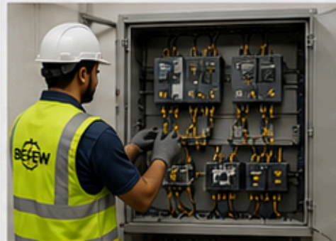
DG SYNCHRONIZATION PANEL INSTALLATION
