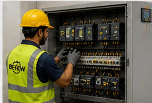
AUTOMATION PANEL INSTALLATION
