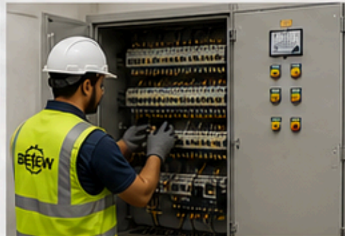
ELDP PANEL INSTALLATION
