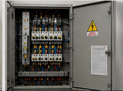
PDB PANEL INSTALLATION
