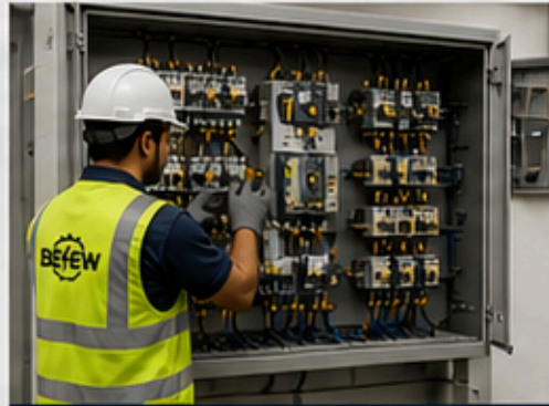
MCC PANEL INSTALLATION
