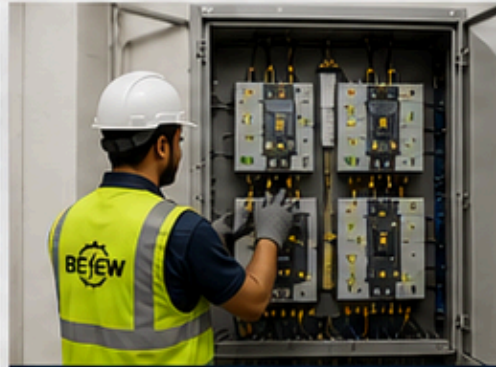
APFC PANEL INSTALLATION
