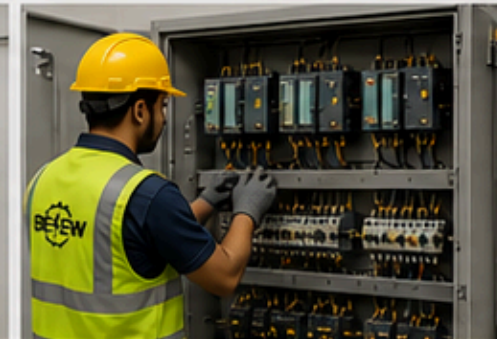
PLC PANEL INSTALLATION
